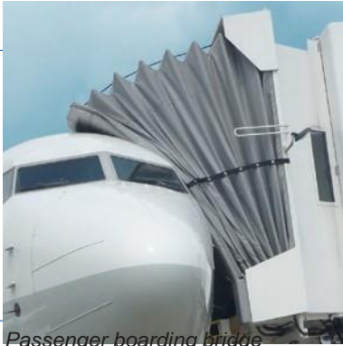
Passenger boarding bridge
